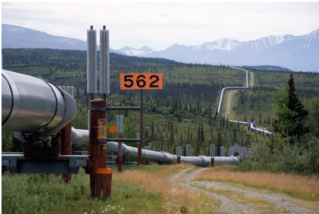
Figure 1.3: Picture of the Trans-Alaska Pipeline. A radiator can be seen in the foreground while the wiggly structure of the pipeline is observable in the background. More details can be found on http://www.alyeska-pipe.com/ and http://en.wikipedia.org/wiki/Trans-Alaska_Pipeline_System .
