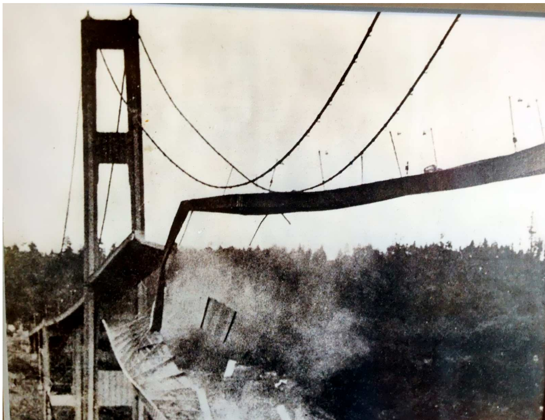
Figure 4.8: Pictures of the Tacoma Narrows bridge on November 7th, 1940 before and during its collapse. After http://en.wikipedia.org/wiki/Tacoma_Narrows_Bridge_(1940) .
